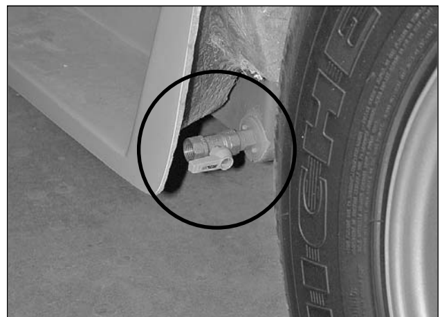
Picture G-P3: Location of the exterior freshwater tank low point drain.
